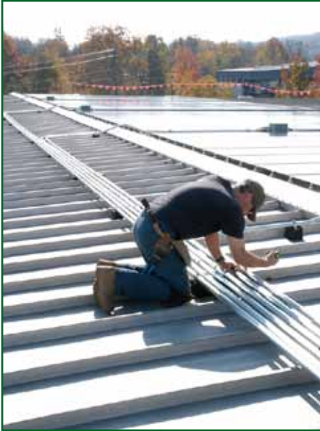
Installation of Siemon's solar power system.
